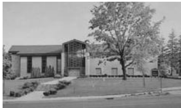
Temple Sholom's old building on Putnam Avenue.
